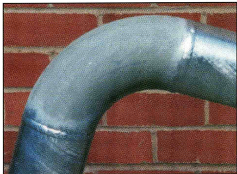
A silicon containing steel (centre) welded to a rimmed or aluminium killed steel (right and left) combines dark and light grey galvanizing.
