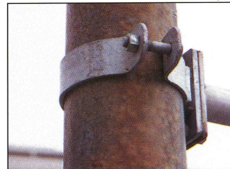
Over thirty years exposure to a mild urban atmosphere - but the steel is fully protected as is shown in the micro-section on the left.
